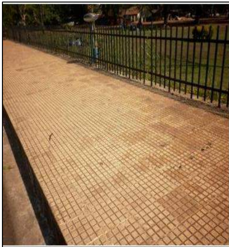
Figure 5-1: Chequered tile on footpath
