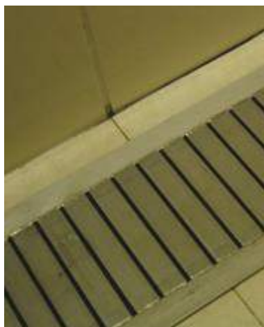
Figure 5-11: Preferred design of gratings
